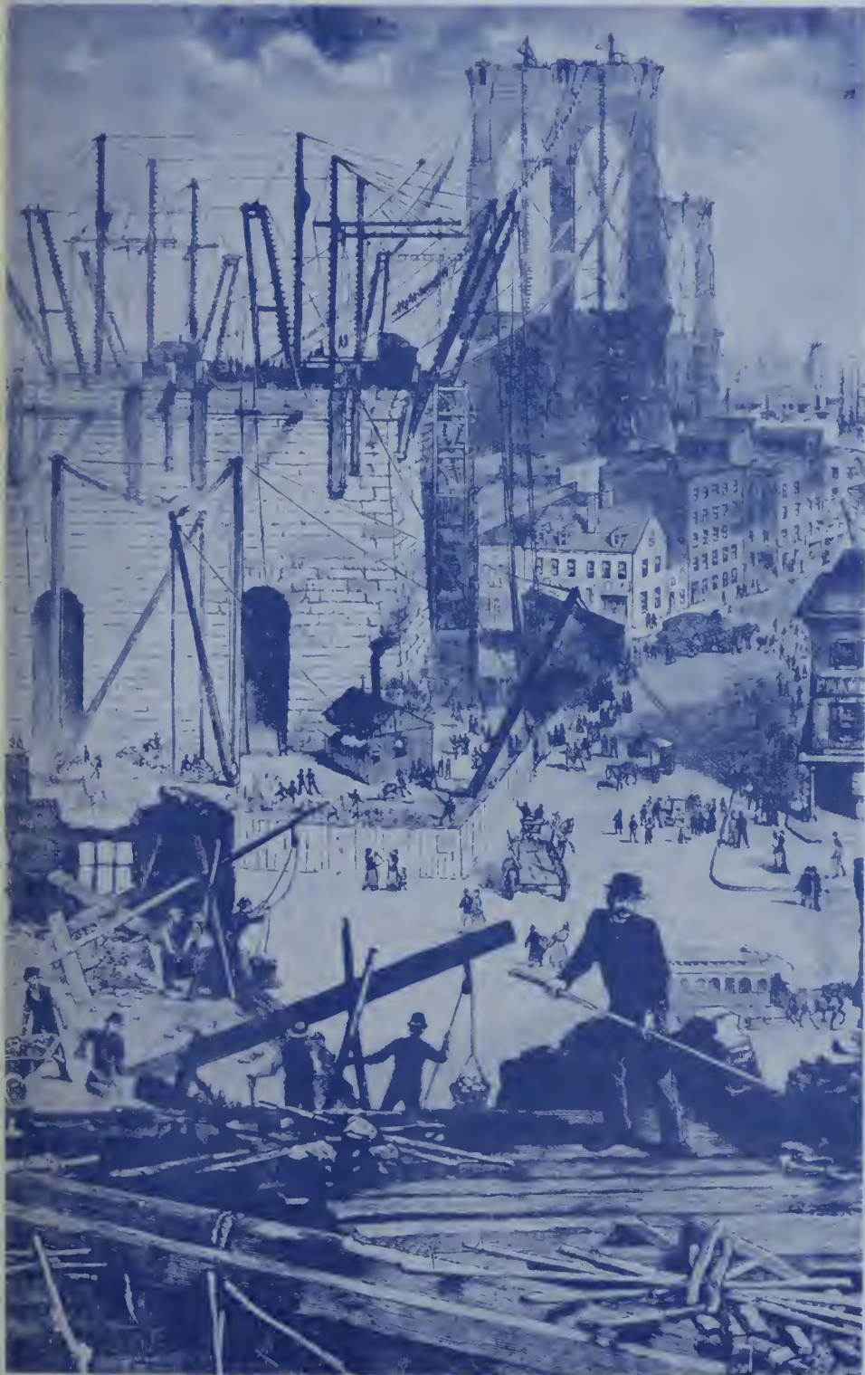
As work progresses on the cables for the bridge—1877—buildings in the way of the New York approach are demolished.
